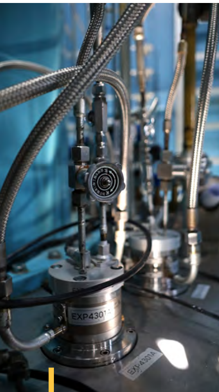
Helium turbine enclosure.
