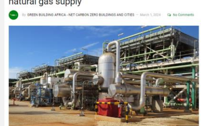
Panda-Temane Complex in Mozambique which supplies SA's petrochemical plants in South Africa. They in turn produce electricity from the gas plus supply the country's industrial gas needs. Image Credit: Sasol
