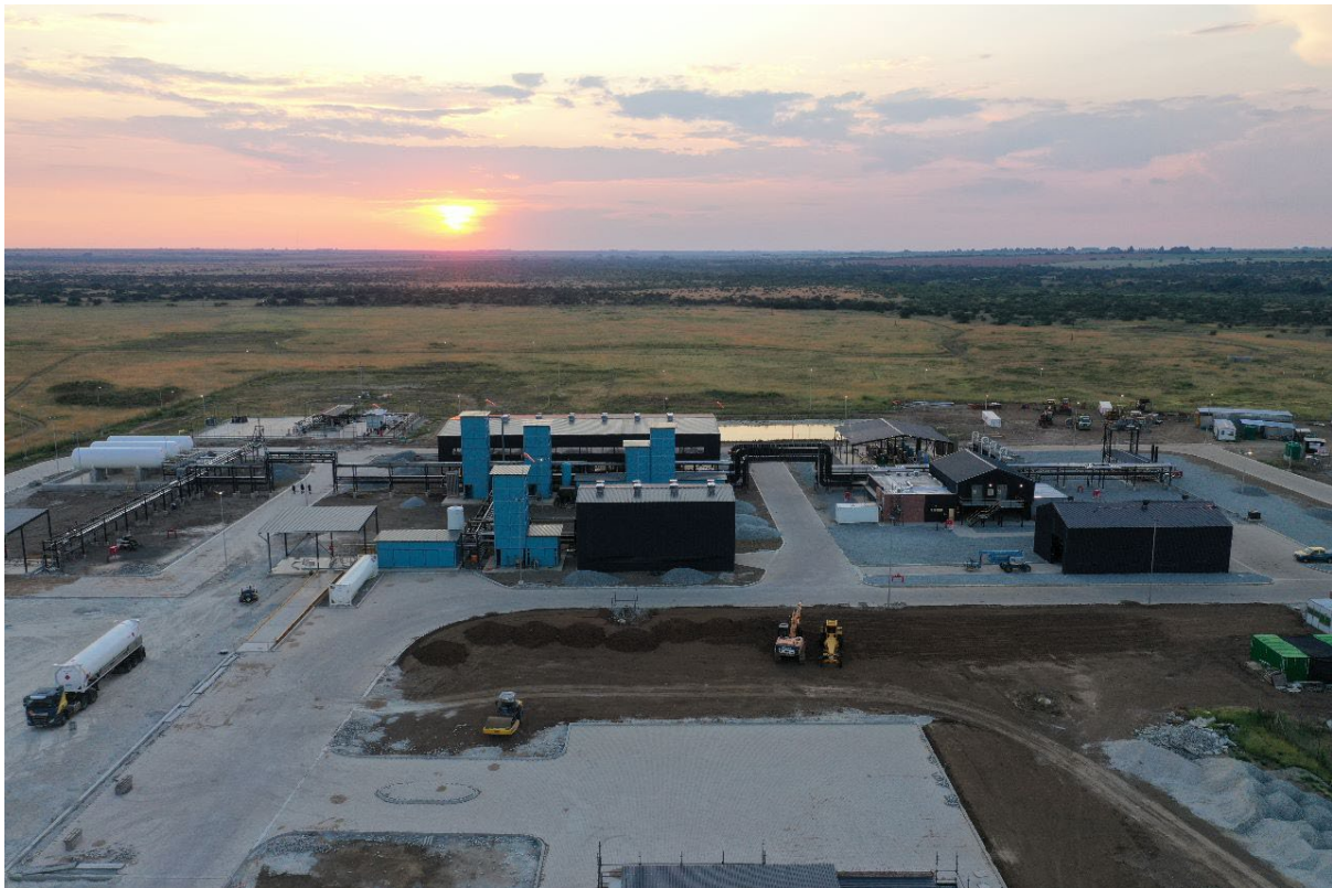
Image: Virginia Gas Plant (helium block)
