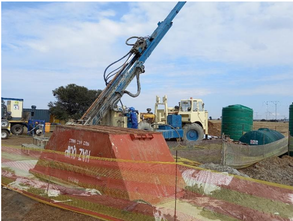
Figure 7: Exploration drilling at well P24b continued.
