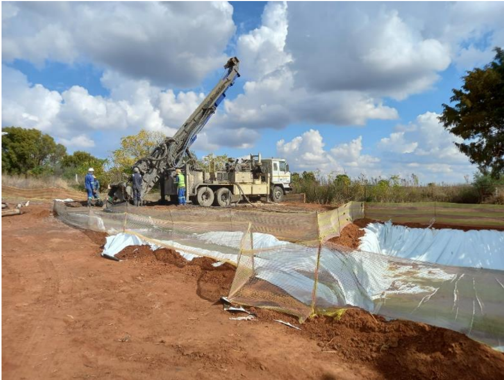
Figure 8: Exploration drilling commenced at well P23.
