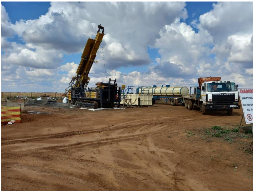
Figure 9: Exploration drilling continued at well P22 continued.
